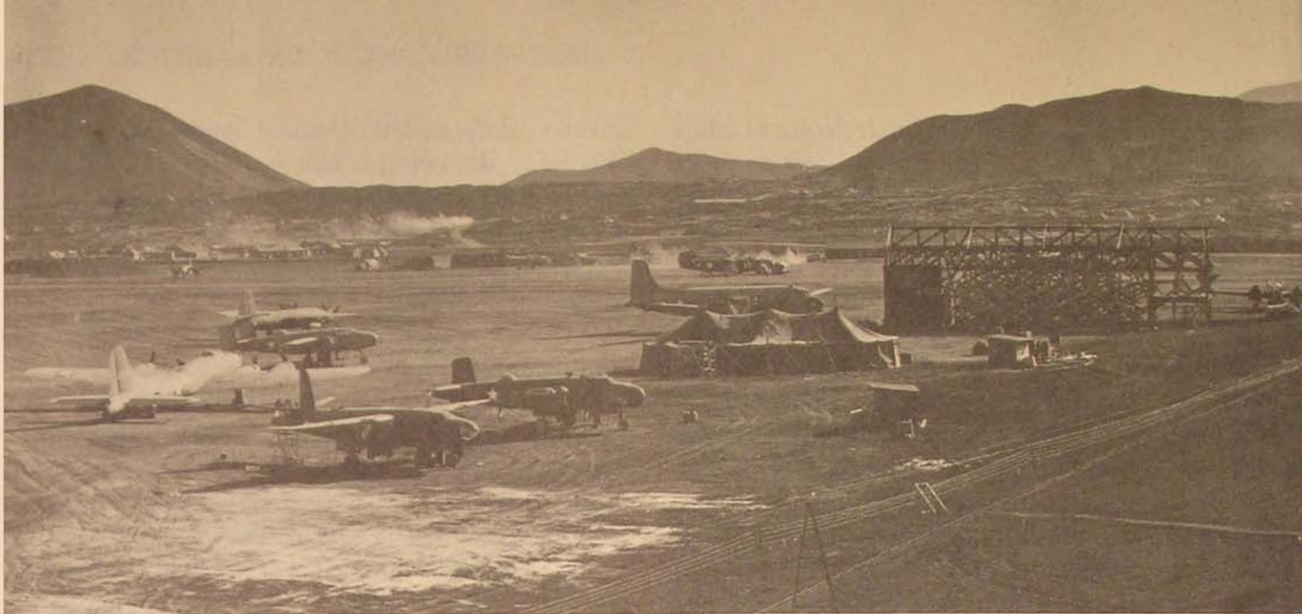
The parking ramp at Wideawake Field welcomed all types. Here, from left to right, the C-47, B-26, B-17, B-26 and B-25 undergoing work on vertical stabilizers, and C-54. In the background a B-24 takes on fuel.
