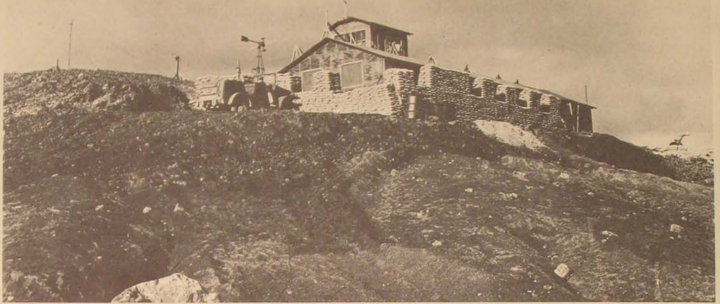
The operations building was on a hill overlooking the runway. Sandbags took account of the possibility of U-boat shellfire.
